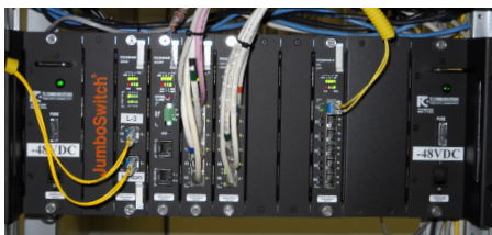
The JumboSwitch 4U chassis at NIPCO’s Central Office currently has four card slots available for future network expansion.
