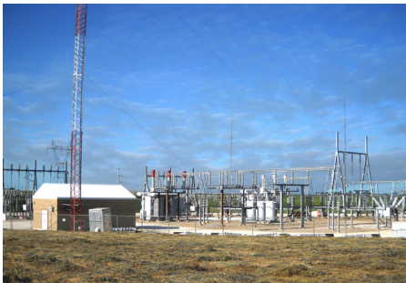
The JumboSwitch in NIPCO's "Eagle" substation connects video cameras, protective relays and a radio link to a remote substation.
