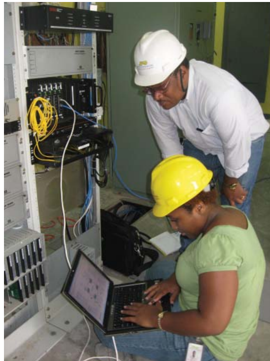
Technician Engineer conducts JumboSwitch network testing.
